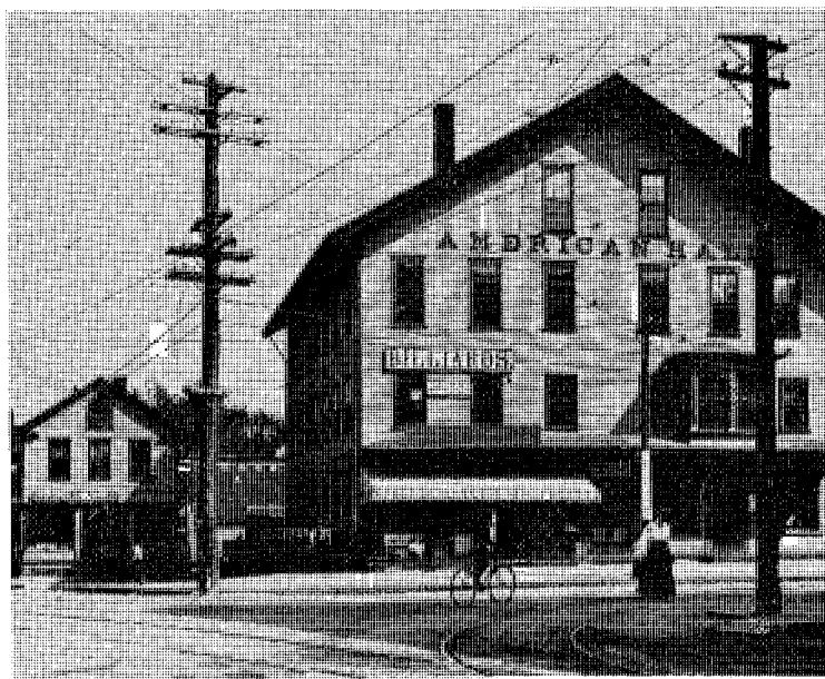
South corner of South Main and Wareham streets. Small building is Peckham's Market. Built about 1850 by George Soule as home and place of business, cabinet maker and undertaker. Peckham's Market was sold in 1924 to George Lang of Onset who operated market until building was demolished in 1933. American Building dates back to the early 1840's and was first occupied by Hon. Philander Washburn's store. In 1854 size of building was doubled, a second story added, called American Hall.
