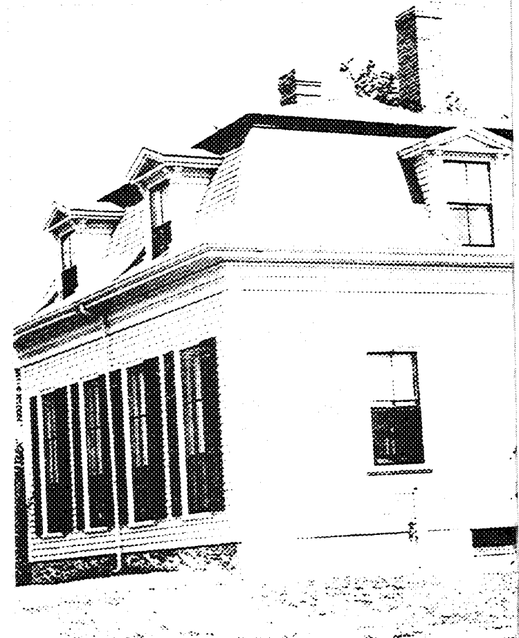
Although commonly employed to give added prestige and a useable third floor to a two-story building, the Mansard roof sits well on a less pretentious structure, as shown at 31 Oak Street; the front windows here being another evidence of "gracious living" in an earlier era.
