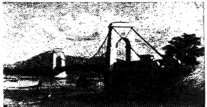
Middlesbrough, England Branch Railway Suspension Bridge 1830
